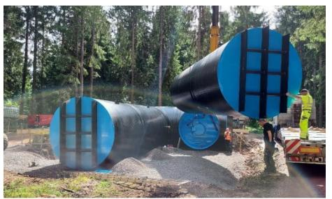
Fig. 5 - Prefabricated container made of PE - 2 x 60 m<sup>3</sup> - Delivery in 3 individual parts
