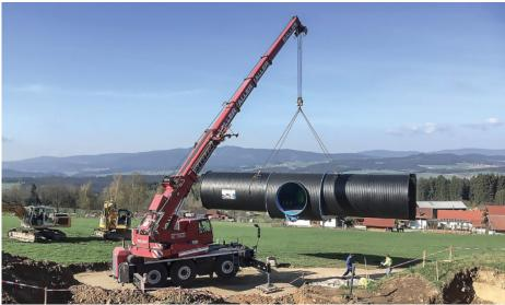
Fig. 4 - PE system container - 2 x 40 m<sup>3</sup> - delivery in one piece
