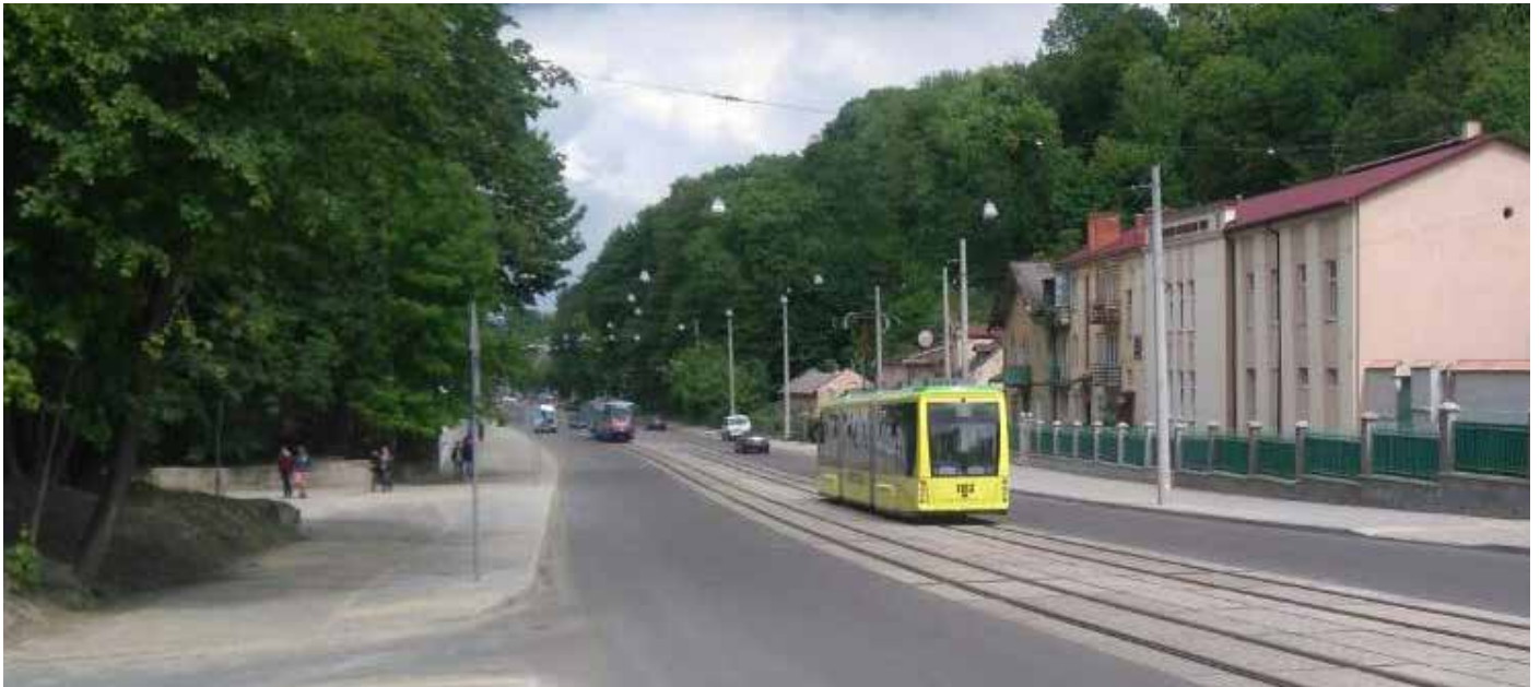
Picture 1: Site after installation
