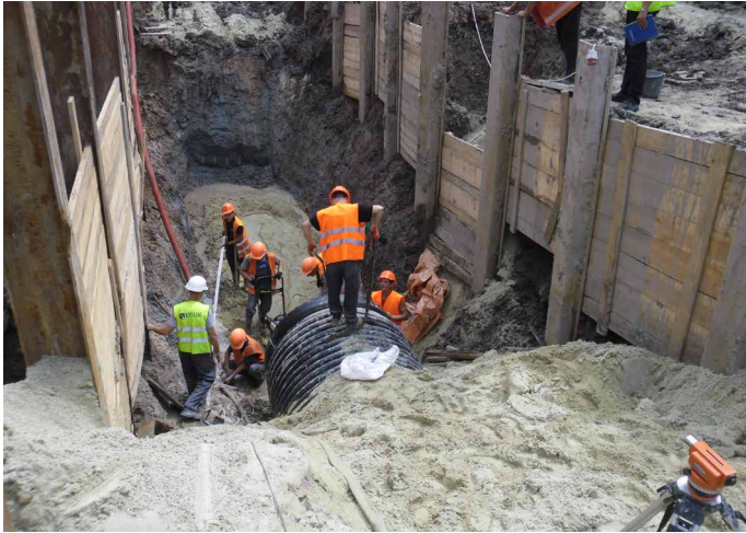
Picture 7: Deep trench installation (until 8m depth)
