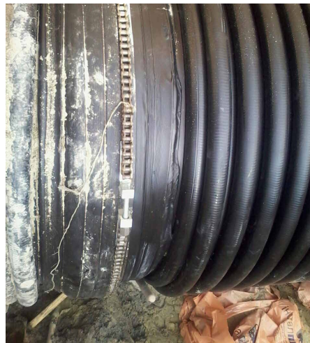
Picture 5: Finished Krah Electrofusion
