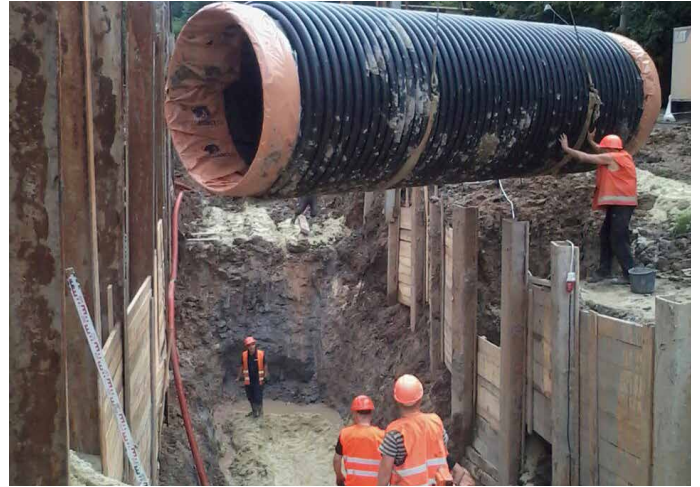
Picture 8: Handling of Krah pipe SN 10, DN 1600 by Instalplast, UKR
