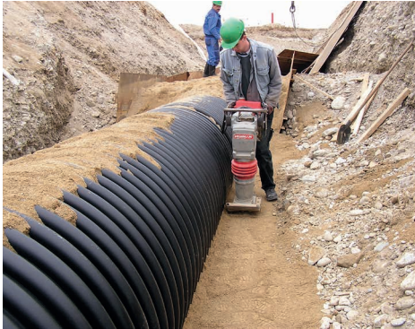
Photo 3: Compaction according to international rules and standards
