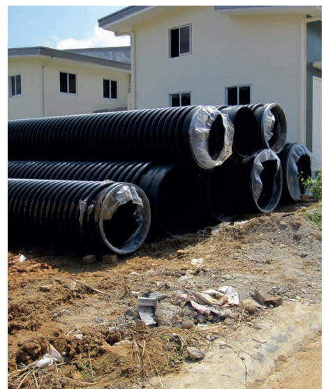
Photo 4: Delivered and staged 800mm diameter Krah profiled wall pipes
