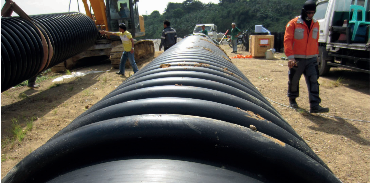
Photo 5: On-going alignment of 1000mm profiled pipes and preparation for electro-fusion jointing.
