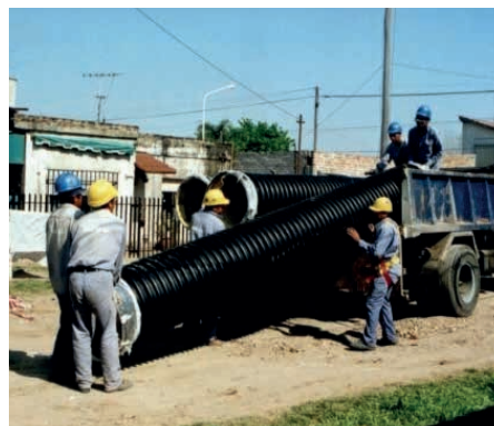
Photo 2: Manual unloading of a Krah pipe
