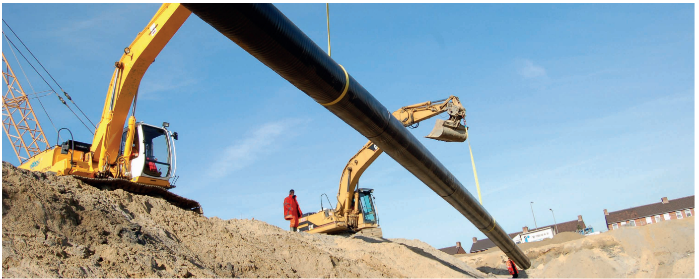
Photo 1: Handling of 24 m pipe string with excavators
