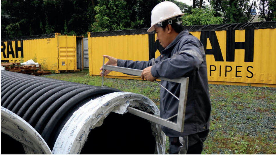
Photo 10: A staff member measuring out the pipe profile
