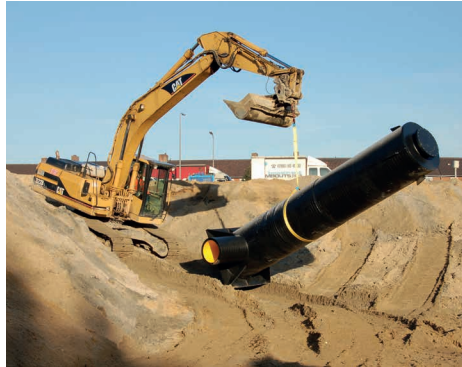
Photo 4: Handling of Krah manhole
