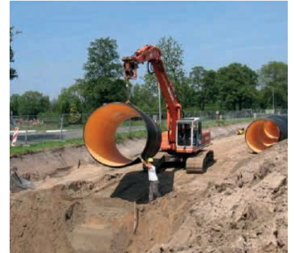
Photo 5: Placing of a Krah pipe
