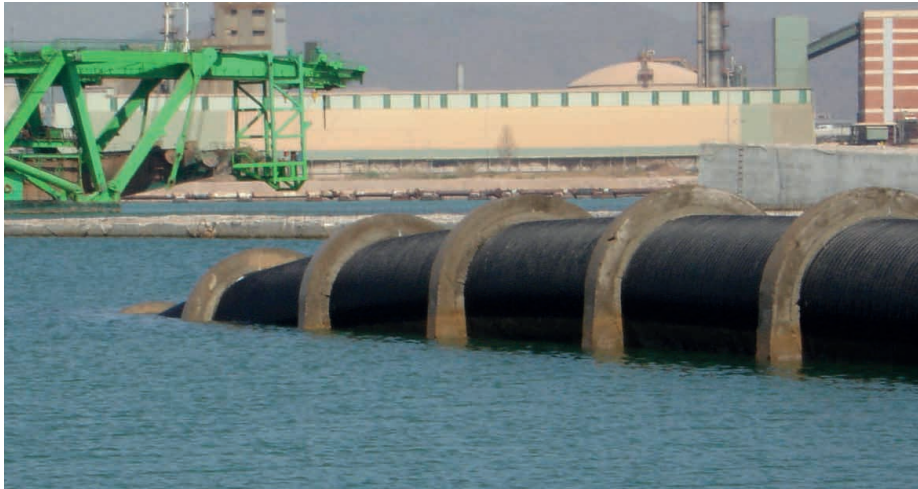
Photo 3: Deployment of a Krah Pipe DN/ID 2400 mm
