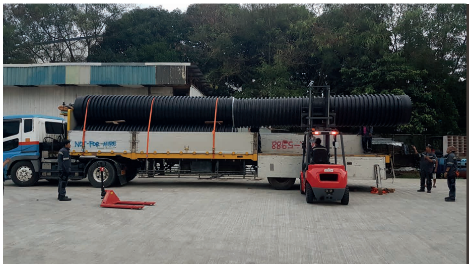
Photo 2: Loading of 1000mm diameter krah profiled wall pipes in a flat bed truck ( 8 pcs of 1000mm diameter pipes and 4 pcs of 800mm diameter pipes of 6m length each)
