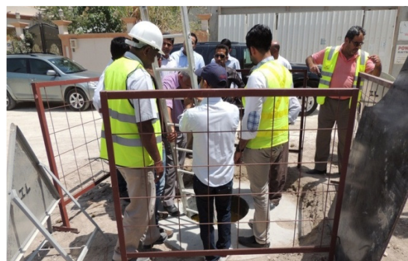
Figure 26: Backfilled to pavement level
