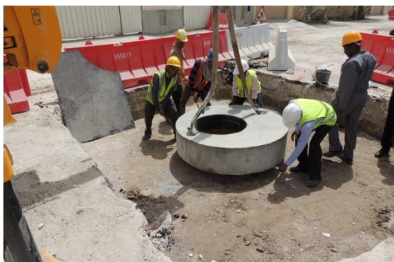
Figure 25: Ready for final road leveling
