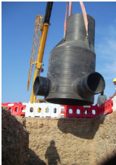
Figure 27: Handling at site
