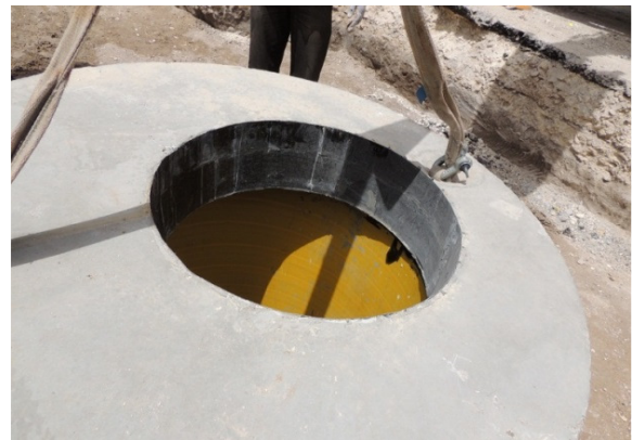
Figure 24: View into Manhole
