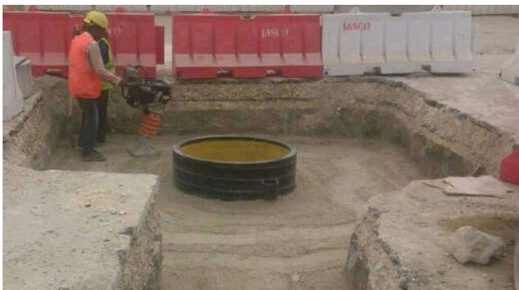
Figure 17: Backfilling & Compaction to 80% of Ground Level
