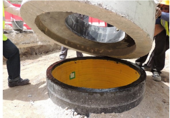
Figure 22: Positioning Top Slab
