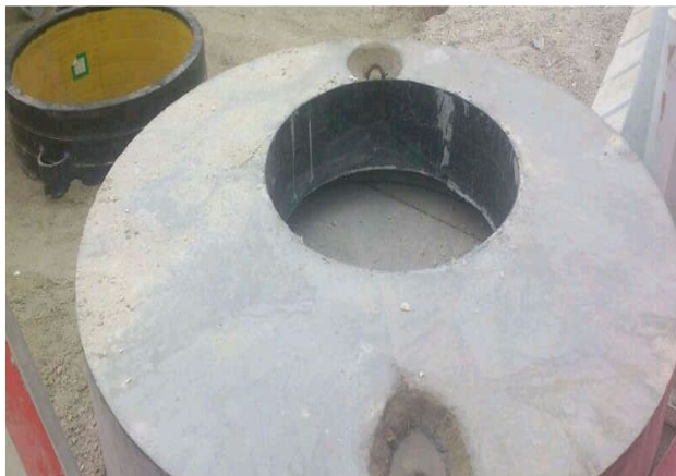
Figure 20: Lined Top Slab
