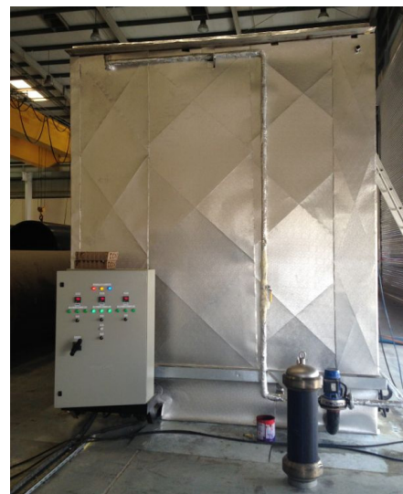
Pic.3: Tank for hydrostatic pressure tests of large diameter pipes and fittings at UGPM Oman
