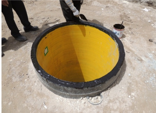
Figure 21: Applying mastic sealant to Manhole Top
