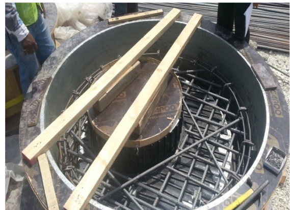
Figure 19: Casting PE liner into Reinforced Top Slab
