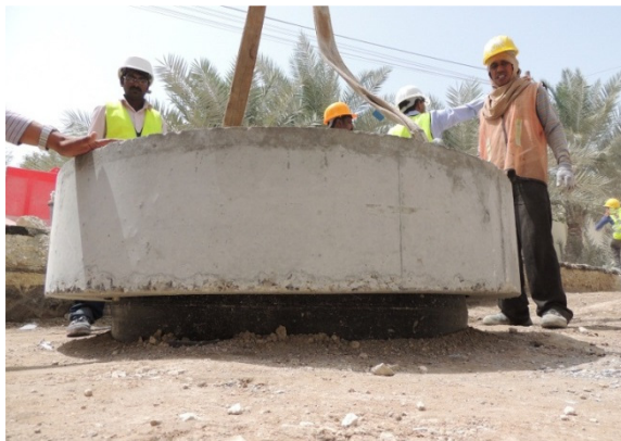
Figure 23: Top Slab positioned onto Manhole
