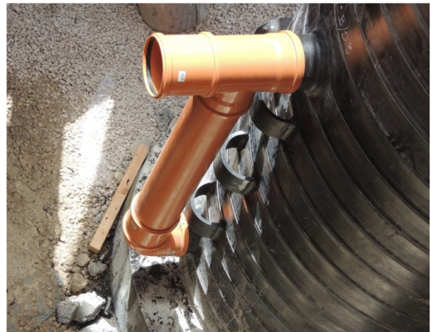
Figure 11: Krah HDPE Manhole – External Backdrop Connection with Grip Rings
