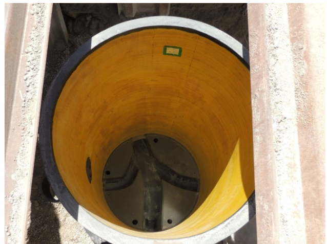
Figure 15: Access holes for pouring of liquid concrete (as required)
