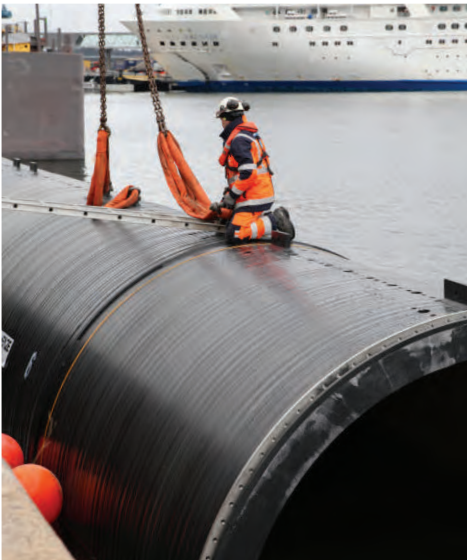
Outfall pipeline DN/ID 3400 mm
