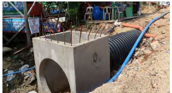
Krah Pipe with a concrete manhole
