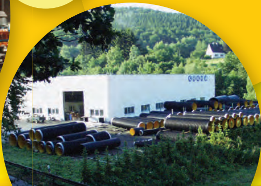
Extension of warehouse and fabrication hall
