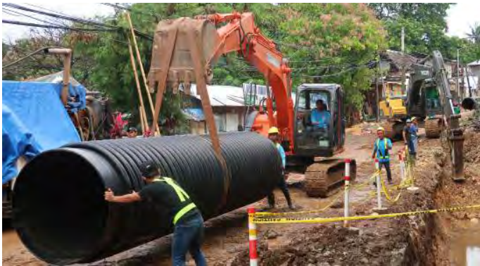
Transporting large Krah-Pipes with light equipment
