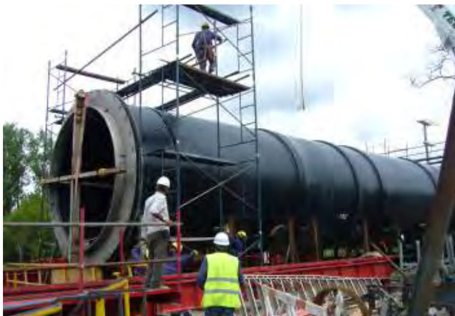
Integrated stub-end for flange connection
