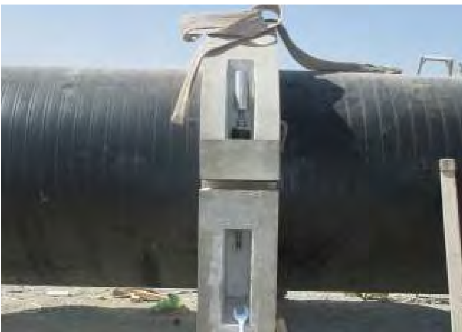
Concrete blocks, mounted in the pipes
