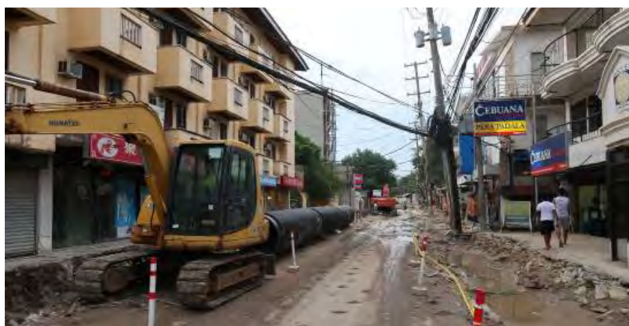
Little streets with big pipes
