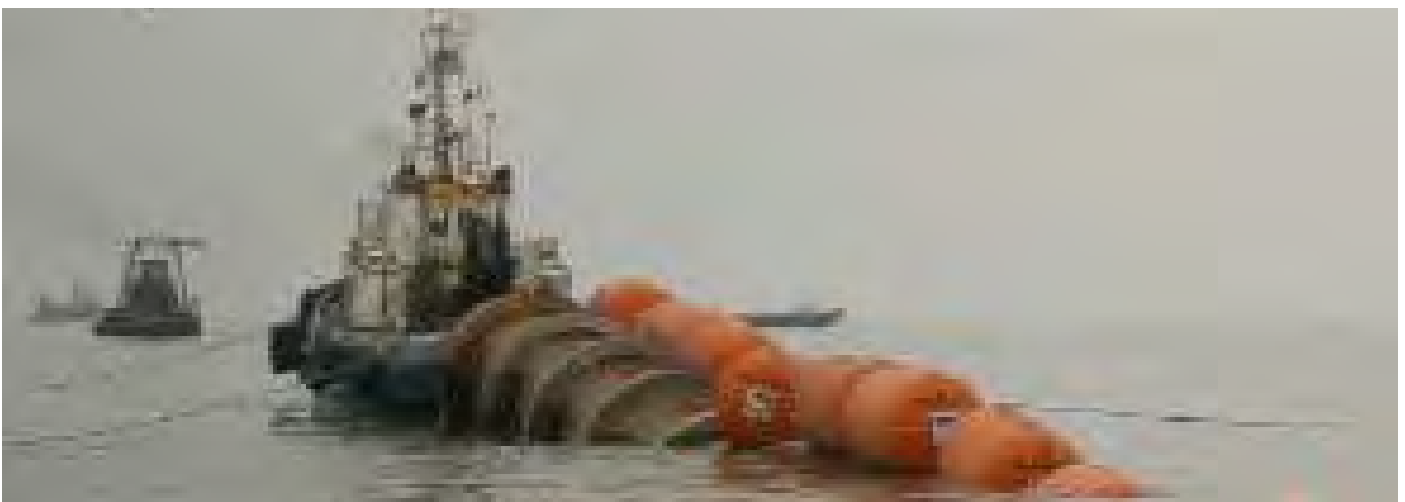
Floaters used during the deployment by PPA&Krah in a project in Peru
