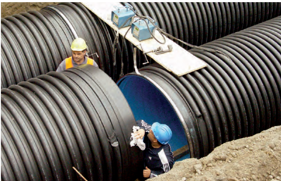
Electro-fusion jointing of big pipes
