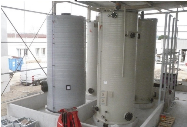
Pic.1: HENZE Double Walled Tanks for the suspension of Bitumen emulsion
