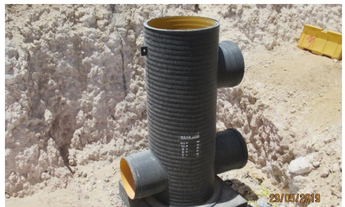
Tailormade manhole design
