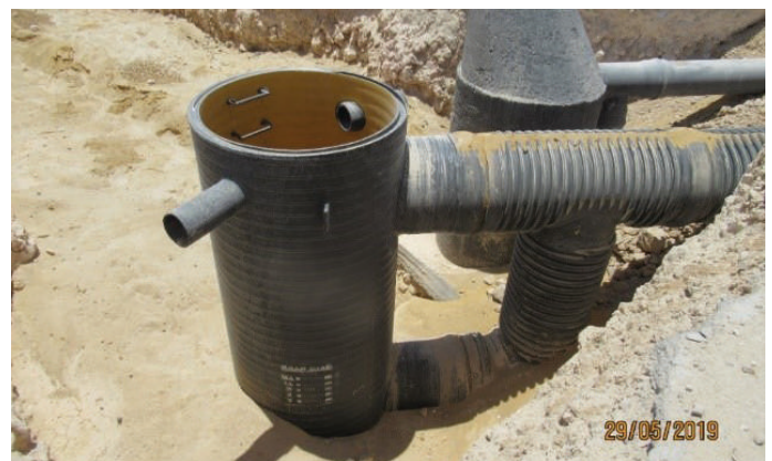
Krah pipe PE100 and concrete manhole in direct comparison
