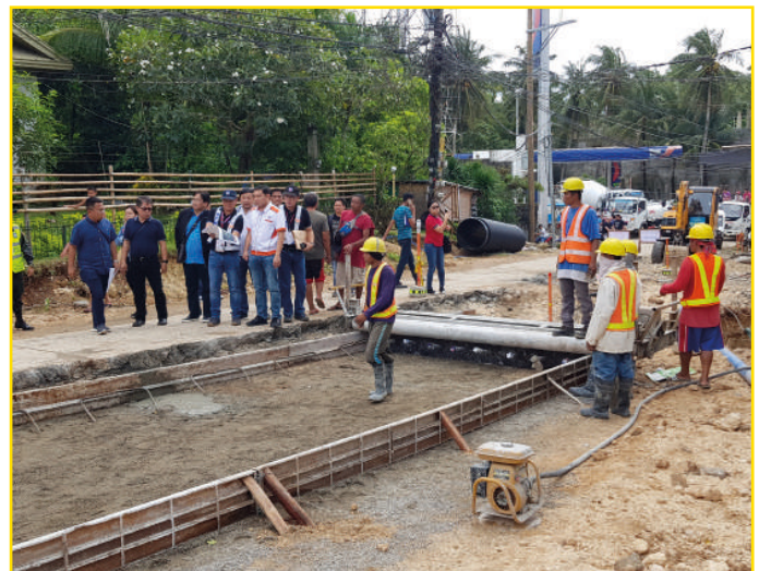
Installation and placement of the pipeline in the streets of Boracay
