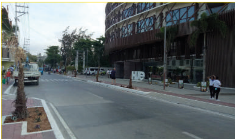
New roads in Boracay with Krah pipes as drainage in both sides
