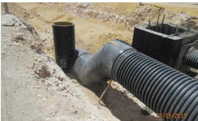
S curve back drop connected to tangential manhole
