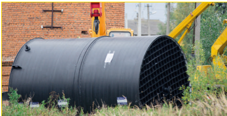
Fig. 2. Installation of the reservoir
