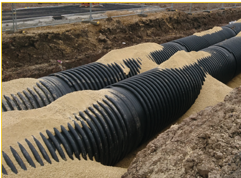
Pipe installation at Wynyard Park
