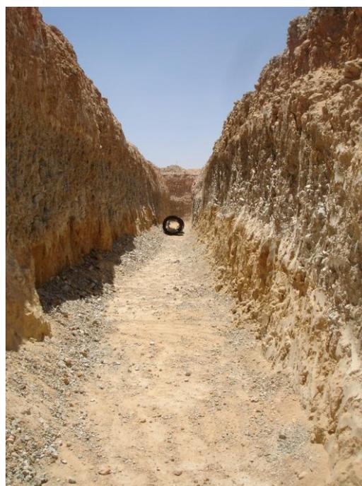
The complete pipeline of length: 3 Km divided between 500, 800 and 1000 mm pipe diameters. The durable welded joint was made by Krah welding equipment simultaneously with the pipe installation in less than half an hour. Thus the construction process was not disturbed and the installation time could be reduced to a minimum. Per day and welding machine more than 60 meters were installed.
