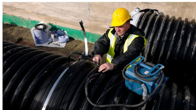
*Joining the 1050 mm diameter pipes by electro-fusion*
