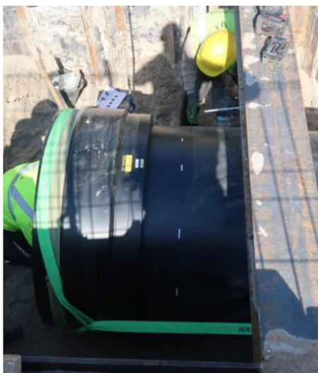
Fig. 9 - Mounting the heating coil sleeve
