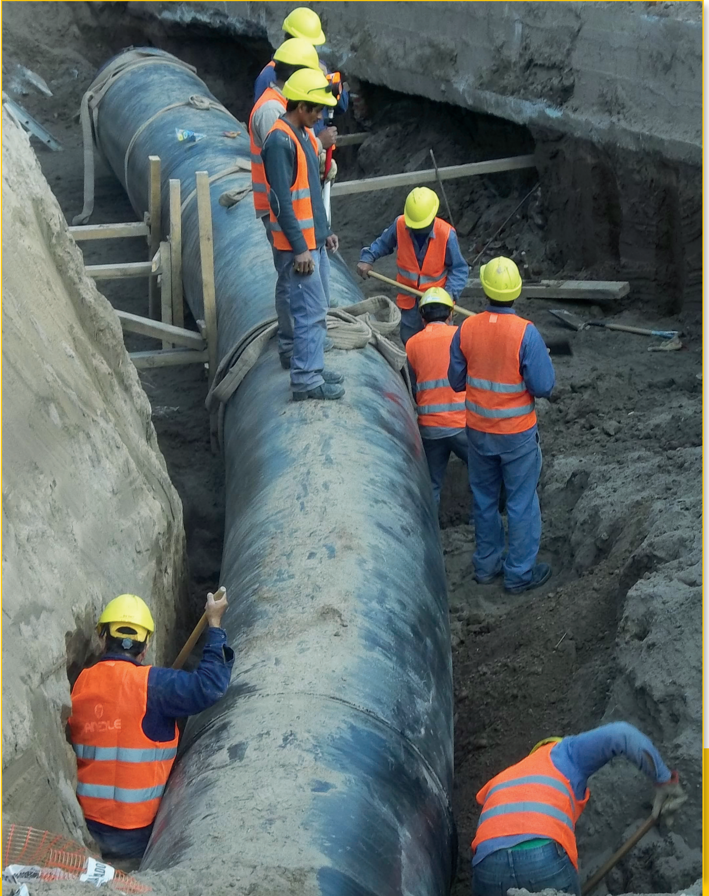
Krah pressure pipes, made of PE 100, during installation.
