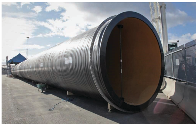
Welding to pipe-strings of 45 m
