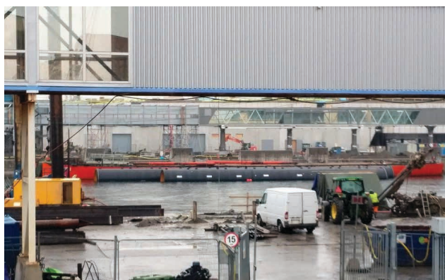
Pipes prepared for concrete-filling of the profiles
