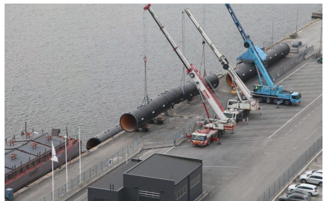
Lifting pipes into the sea
