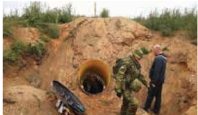
A buried pipeline used as access tunnel and bomb shelter
