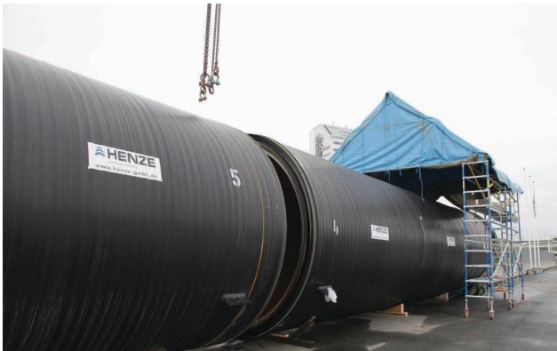
Joining Pipes by using KRAH Electrofusion
