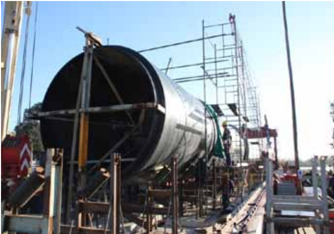
Fixing of the steel cross
