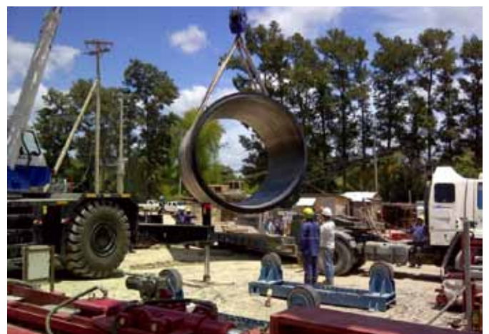
Pipe transportation on the construction site
