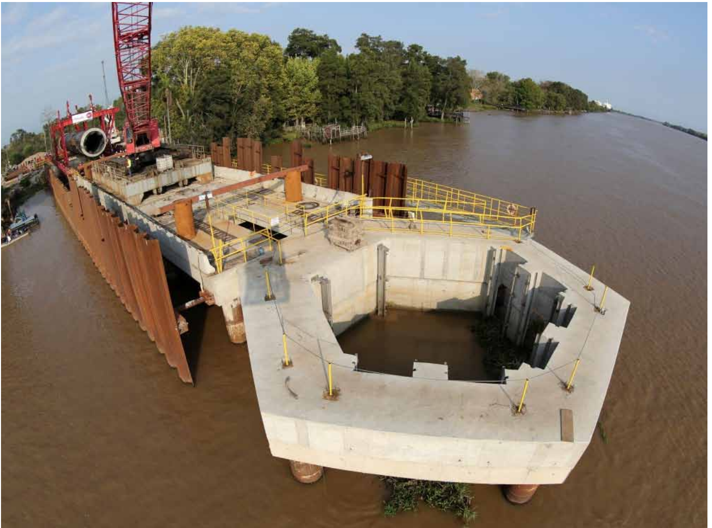
Concrete basin, river side
