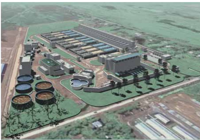
Overviews of water treatment plant in Tigre, Argentina (Aguas del Paraná)
