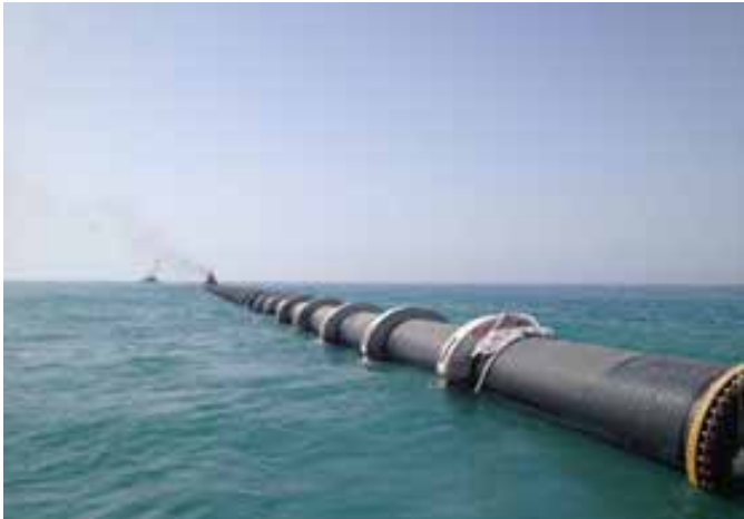
Launching pipe string
