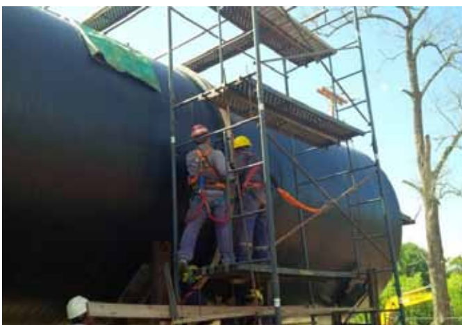
Two pipes being connected
