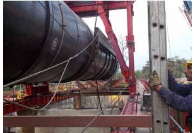
Welded pipe line right before the sinking procedure
