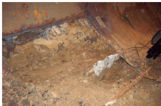
Inside surface of the original pipeline
