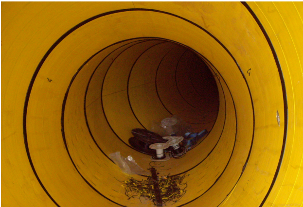
Installing of 1250mm segments into the closed pipeline under the transformers
