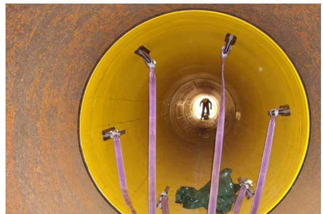
Stubs for anchoring the pulling ropes and spreading pulling loads
