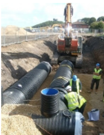
Instaling of 114 metres of Ridgistorm-XL pipe in 1050 mm diameter
