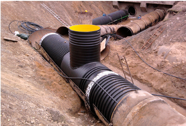
E-fusion connected pipe with integrated pressure manhole to the main pipeline
