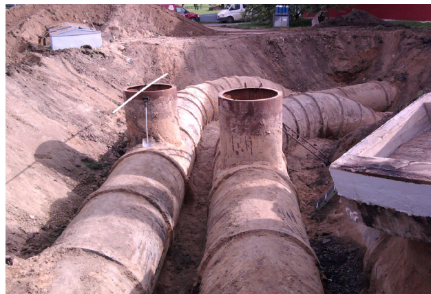
Original pipelines exposed
