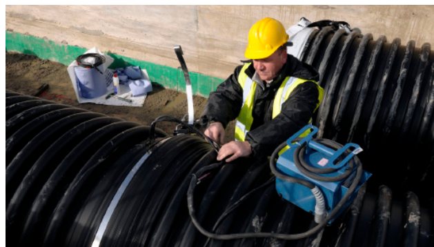
Joining the 1050 mm diameter pipes by electro-fusion
