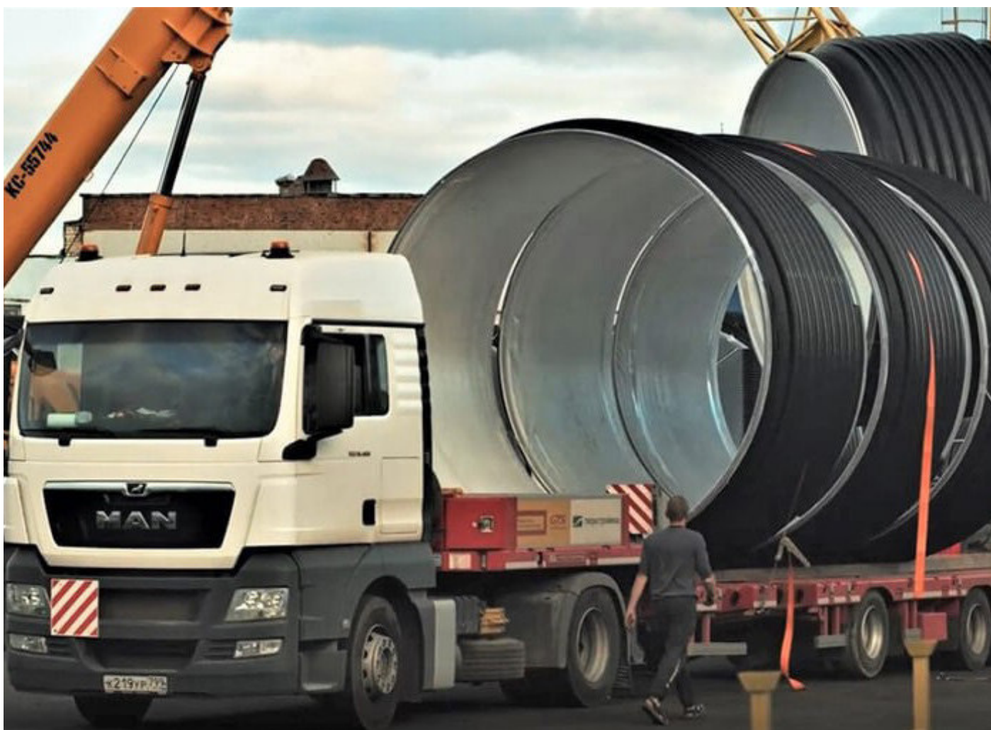
Loading the pipes onto the truck
