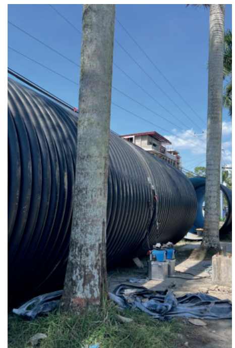
Pre-jointing of DN/ID 3000mm Krah pipes along Tagum rd.
