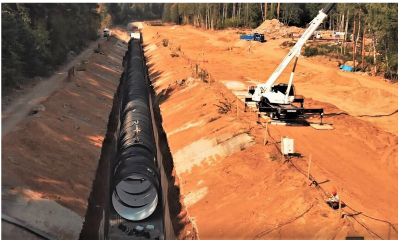
Installing the pipes in the trench
