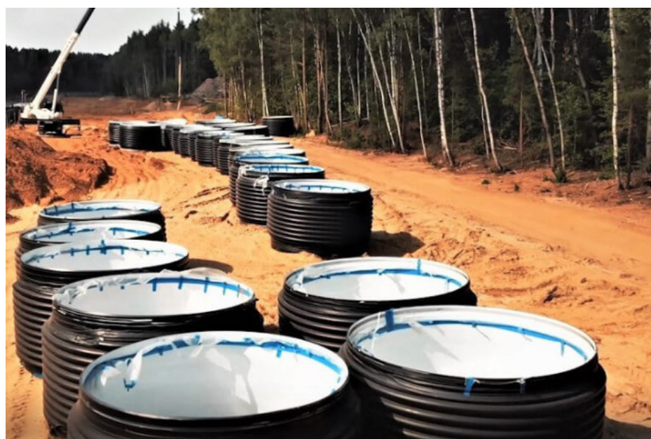
Pipes ready for installation
