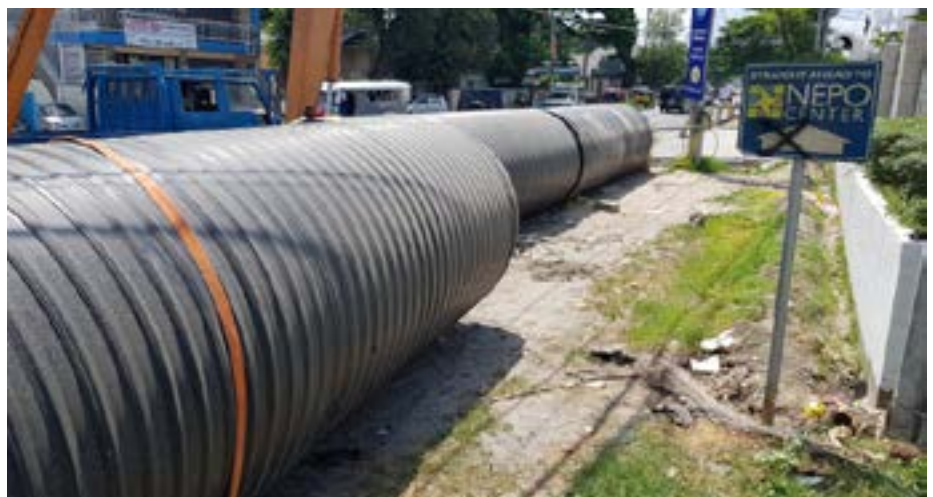
Pic. 5: Before installation
