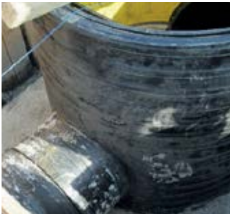
Pic 3: Krah stormwater manhole installation
