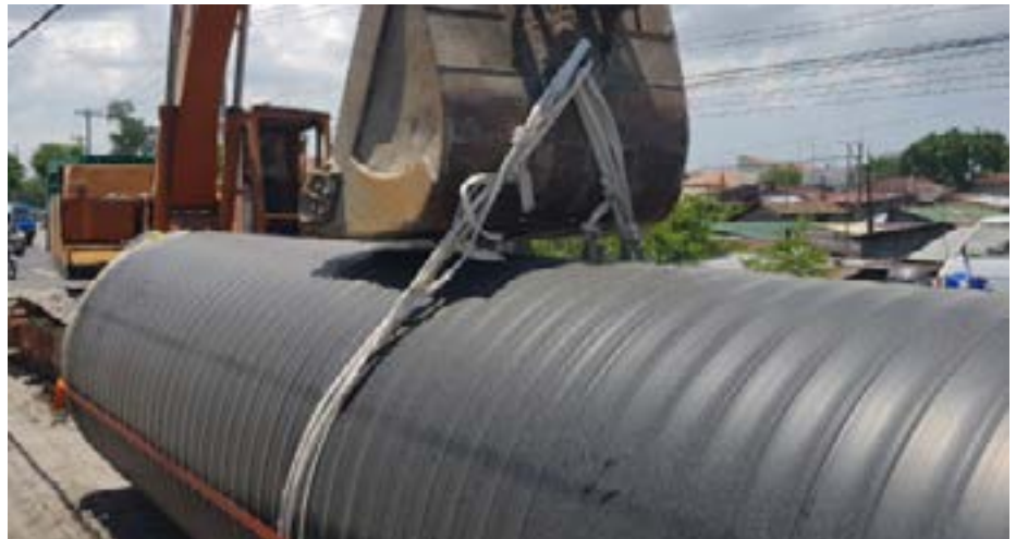
Pic. 4: Lifting Krahelectrofusion pipes with an excavator
