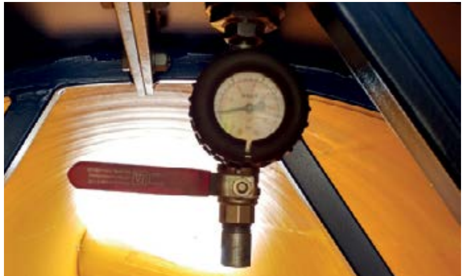
Pic. 2: Tightness test on a Krah pipe
