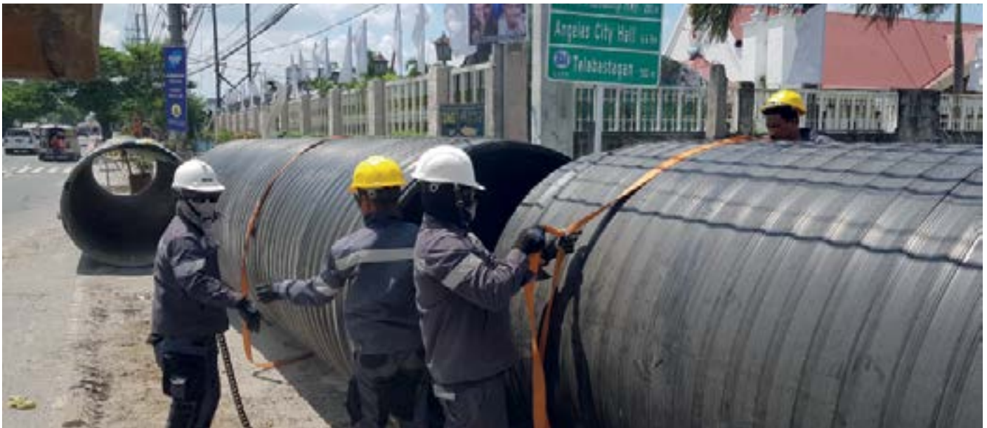
Pic. 1: The Krah team installing the pipeline
