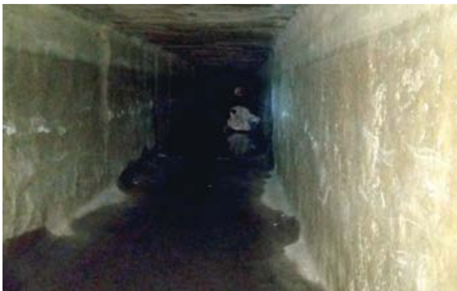
Pic. 1: Underground water conduit to be reconstructed
