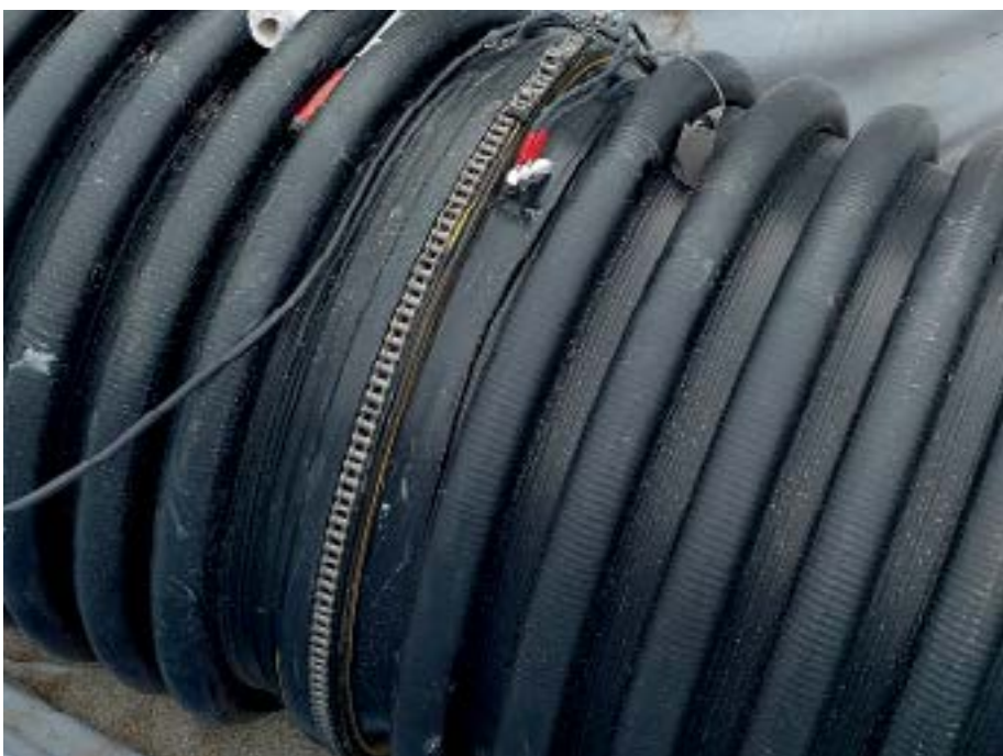
Pic. 3: Electrofusion joint carried out on a Krah pipe
