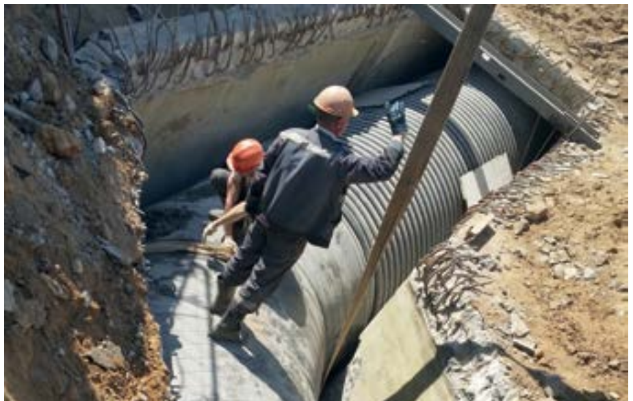
Pic. 3: CORSYS PLUS bending connection in open conduit
