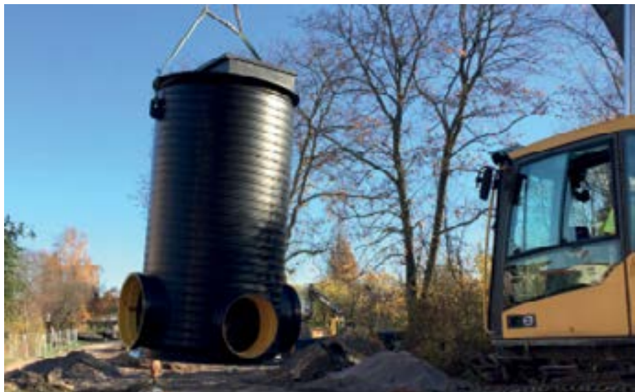
Pic.2: Krah Pipes Manhole
