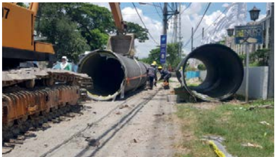
Pic. 2: Arrangement of Krah pipes
