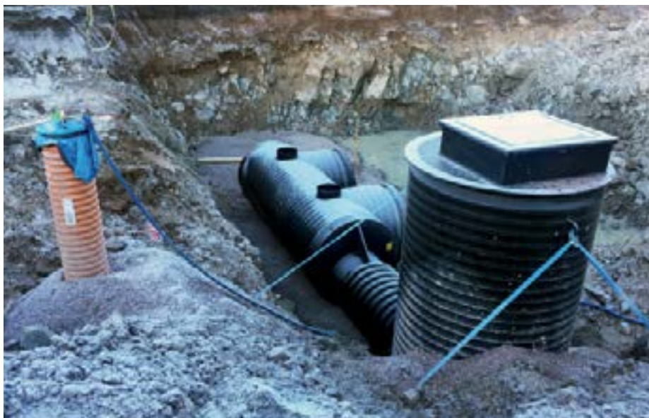
Pic.1: Sewage collection tank during installation
