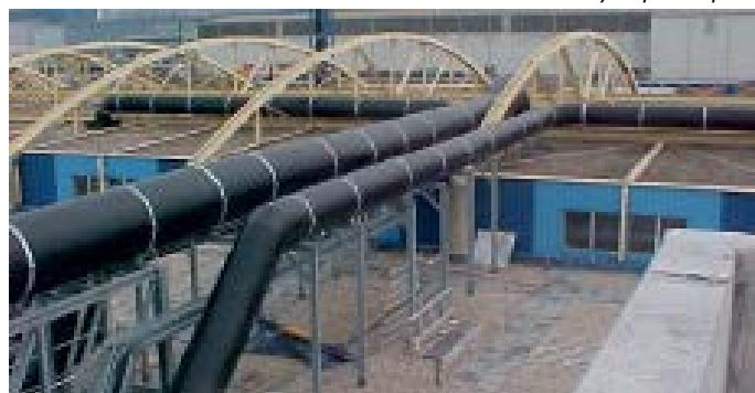
Picture 4: Roof installation of Krah pipe ventilation, PE 100, DN/ID 800 - 1400 mm
