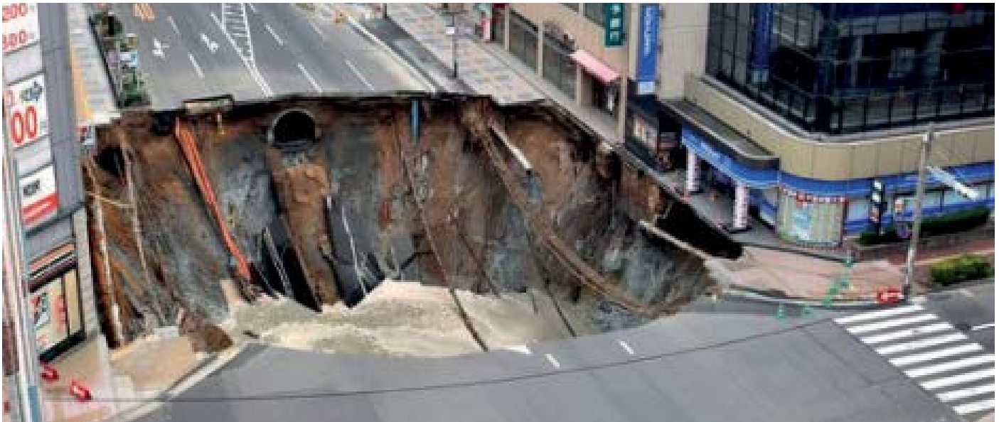
Pic. 4: Repairing a sinkhole sewage line with Krah-Pipes – within 48 hrs.
