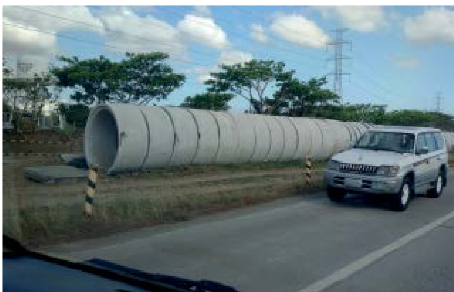
Pic. 2: Concrete pipes with many connections (Source: Krah Pipes GmbH & Co. KG)
