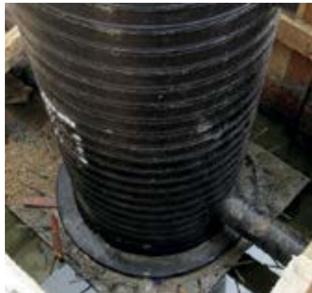
Pic 4: Krah sewage manhole installation
