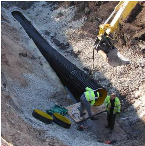
Pic. 3 – Preparation for the welding of two segments
