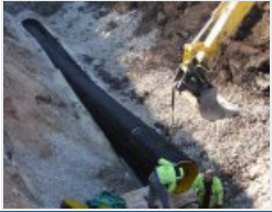
Tartu Ihaste DN1500 Pipeline Renovation Project
