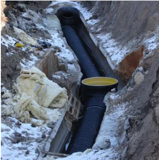
Pic. 6 – Manhole ID1500
