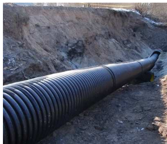
Pic. 5 – Pushing pipe segment into the old concrete pipeline
