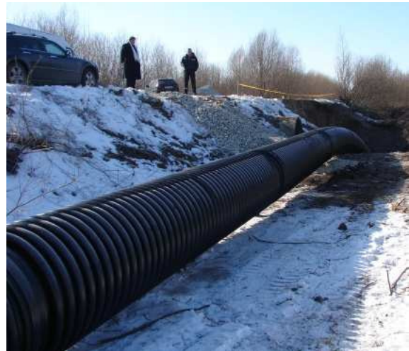
Pic. 4 – Pushing pipe segment into the old concrete pipeline
