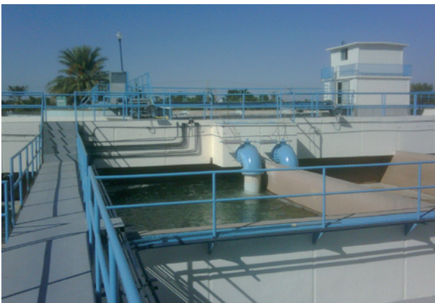
South Water Treatment Plant in Obregon Sonora
