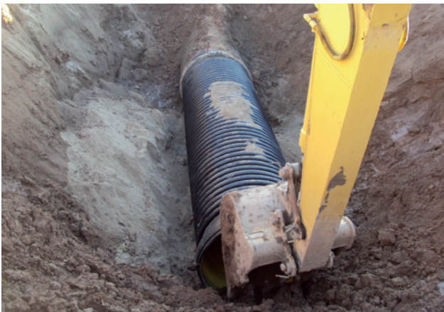
Pipe Installation
