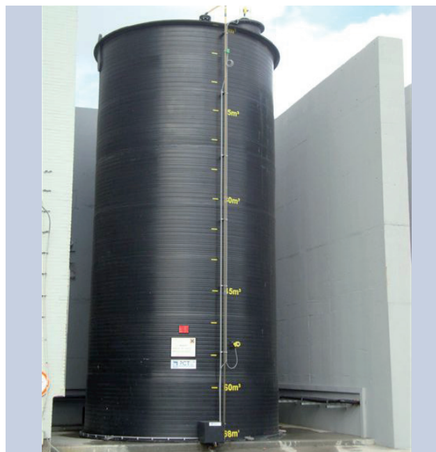
Storage tanks 68 m 3 , manufactured by PCT, Belgium design acc. DVS 2205
