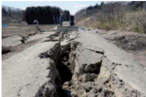
The length of cracks is 1.4km in succession. Depth of crack is 1.6m between top of pipe to ground level. Joints are deformed so much.
