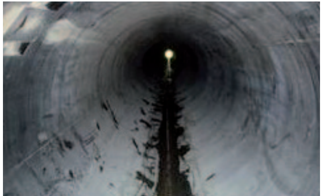
Osaki city Miyagi Pref. 1200mmID , Total length are 60m. We didn't have any damage of appearance with naked eyes. Maximum deflections are 3.3% in upstream area
