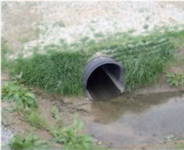
Osaki city Miyagi Pref. 1200mmID , Total length are 60m. We didn't have any damage of appearance with naked eyes. Maximum deflections are 3.3% in upstream area
