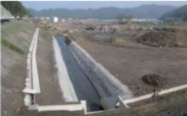
Osaki city Miyagi Pref. 1200mmID , Total length are 60m. We didn't have any damage of appearance with naked eyes. Maximum deflections are 3.3% in upstream area
