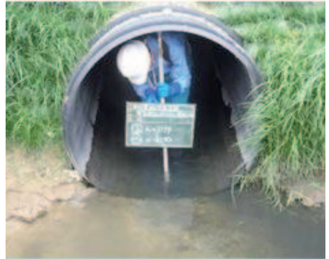
Osaki city Miyagi Pref. 1200mmID , Total length are 60m. We didn't have any damage of appearance with naked eyes. Maximum deflections are 3.3% in upstream area
