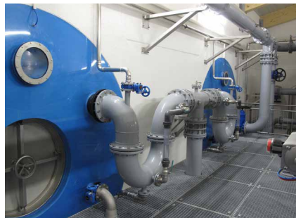
Pic. 5 : Finished waterworks "Vogelhölzle" with building and pipe containers under embankment
