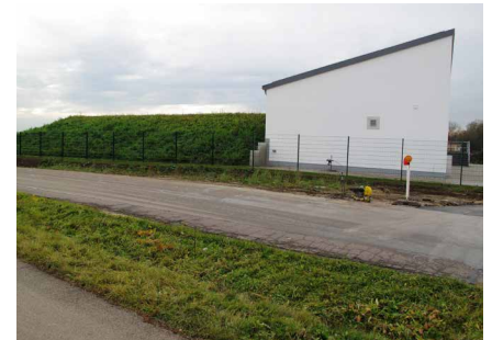
Pic. 4: Functional walls integrated into the plant engineering in the waterworks
