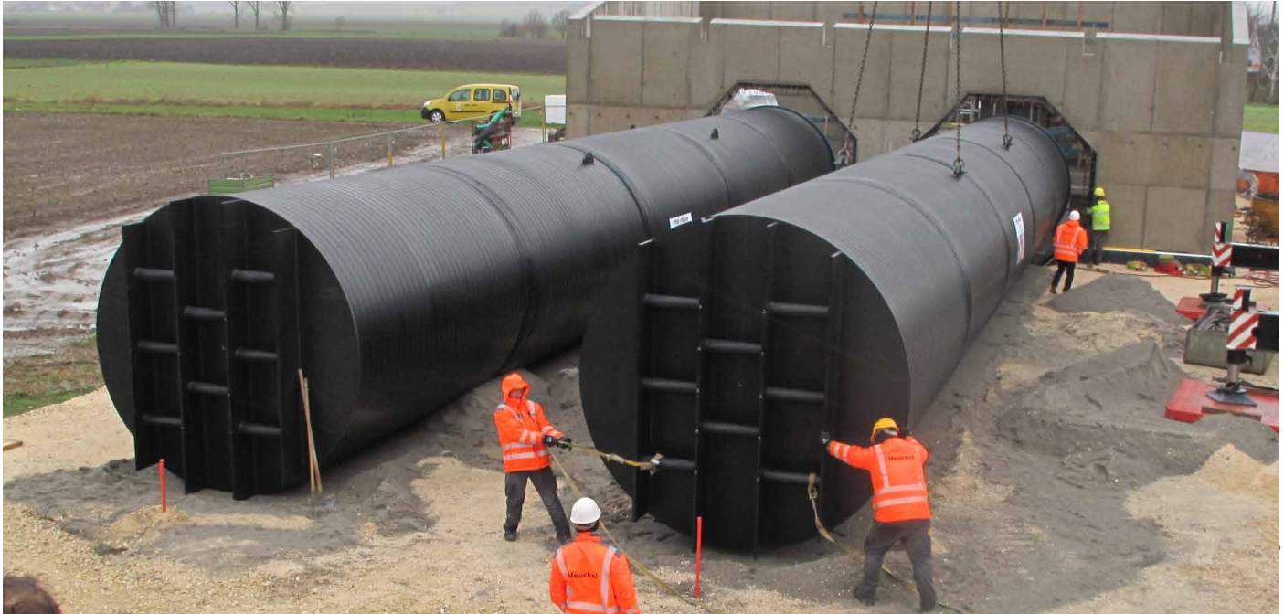
Pic. 2 : Placement of the pipe containers on previously prepared soil
