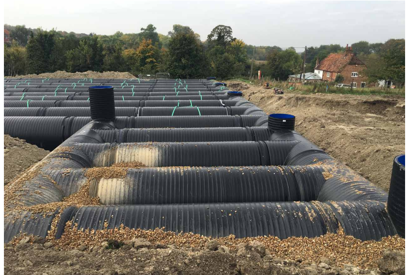
Construction site in Bedfordshire, England
