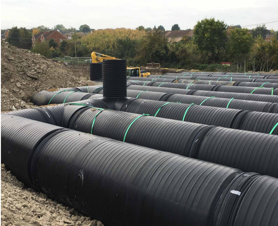
Construction site in Houghton Regis
