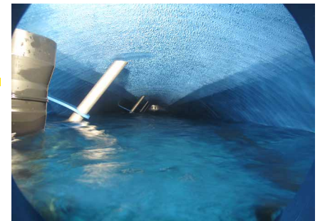
Pic. 6 : View through inspection hole on water surface
