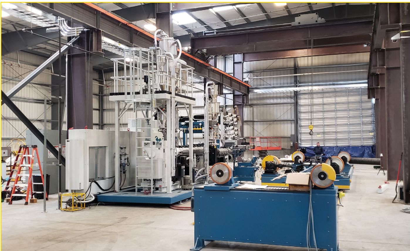
Installing the dismantling station
