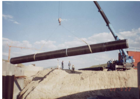
prefabricated pipe length of 30m, with electric fusion socket and spigot end
