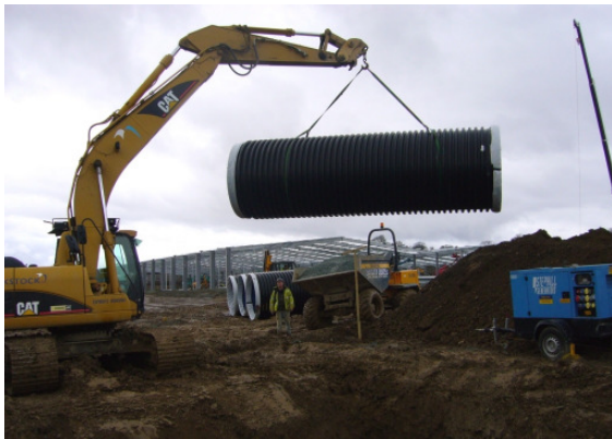
Standard pipe length of 6m, with electric fusion socket and spigot end
