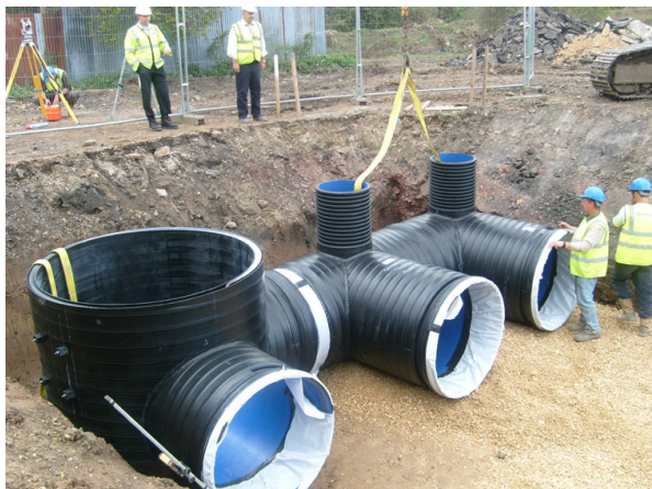
Water retention tank during installation (pipes, manholes, fittings)
