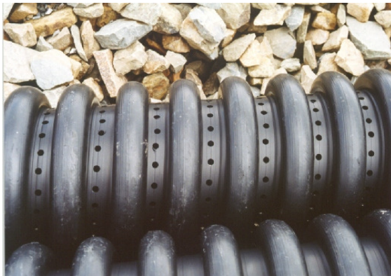
Drainage pipe system
