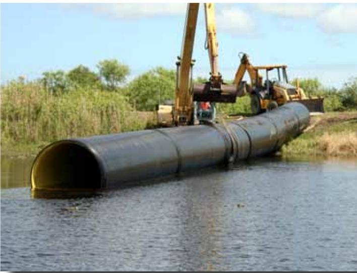
*The electrofused PPT pipe was placed in the water to be submerged under water and pushed into the old pipe.*
