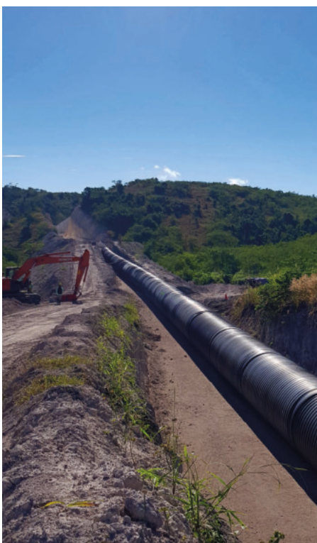
Laying of Krah pipes over sand bedding
