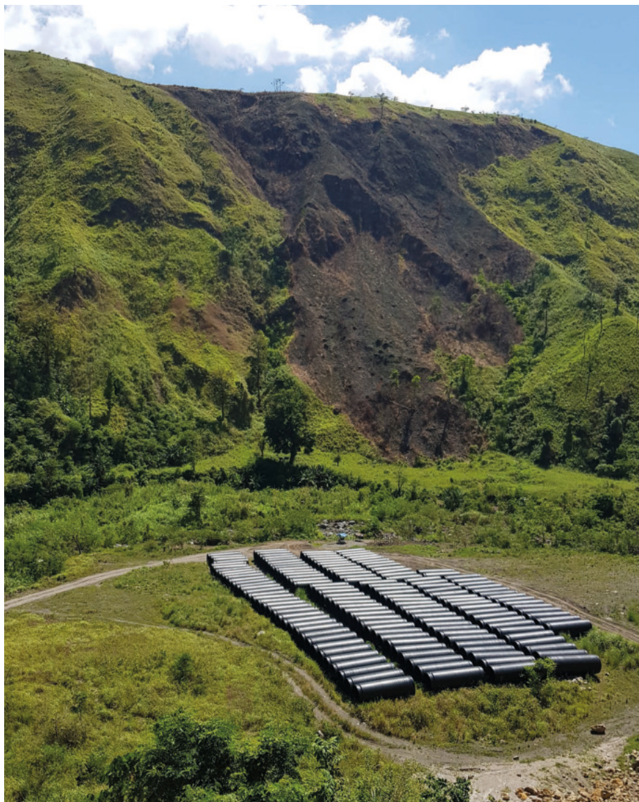
Staging area of DN/ID 2000mm pipes in Sitio Lunay
