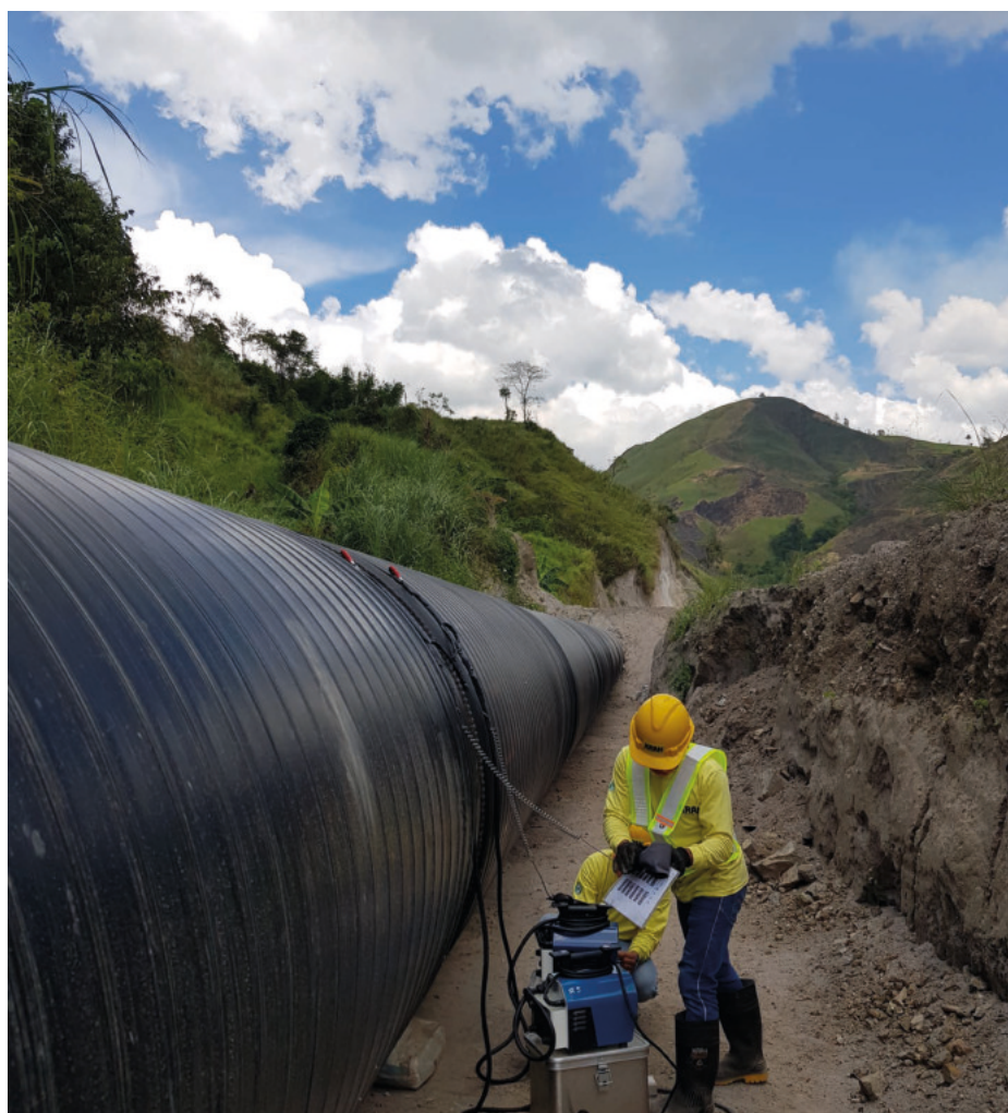
On-going electrofusion jointing of Krah pipes
