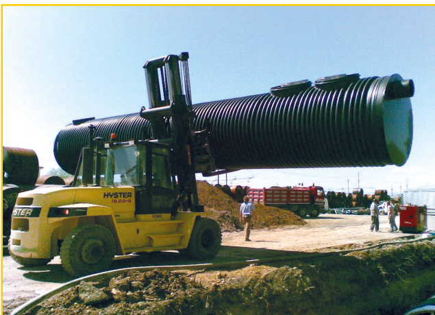
Easy handling of a watertank DN/ID 1800mm (71")
