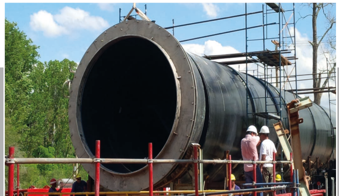
DN/OD 4000mm (158") solid wall pipe with SDR 11
