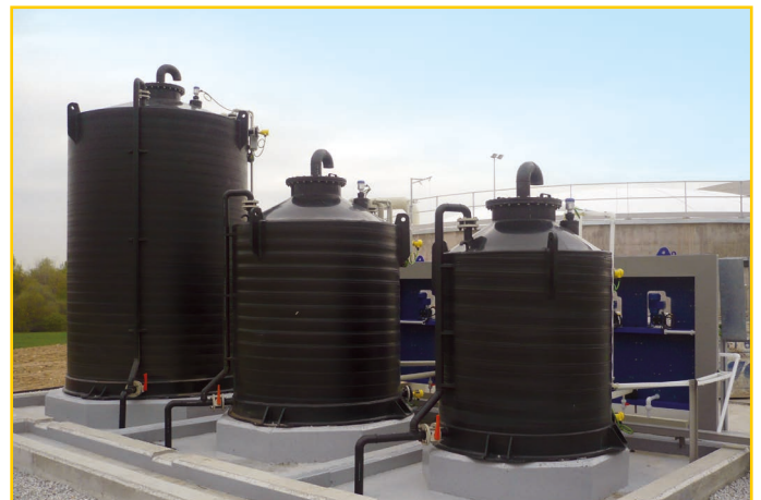
Shafts for landfill
