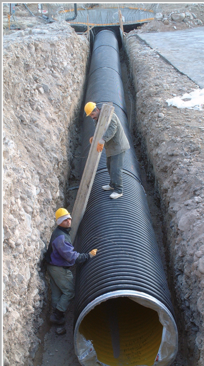
Installation of a Krah pipe in a very narrow trench
