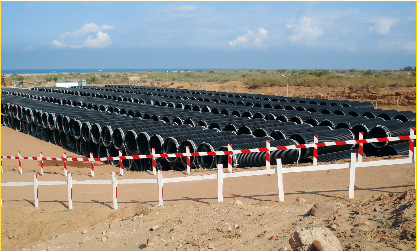
Open storage of pipes DN/ID 1600mm (63")
