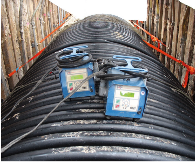
Electro-Fusion joint DN/ID 1800mm (71")
