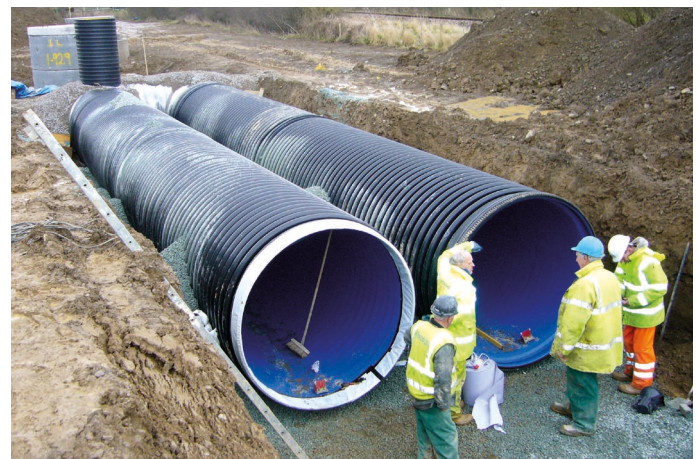
Installation of stormwater system DN/ID 1800mm (71")
