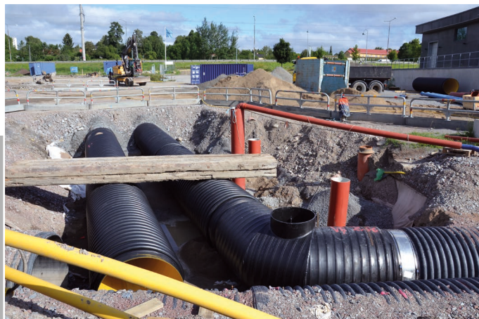
Fire fighting water tank
