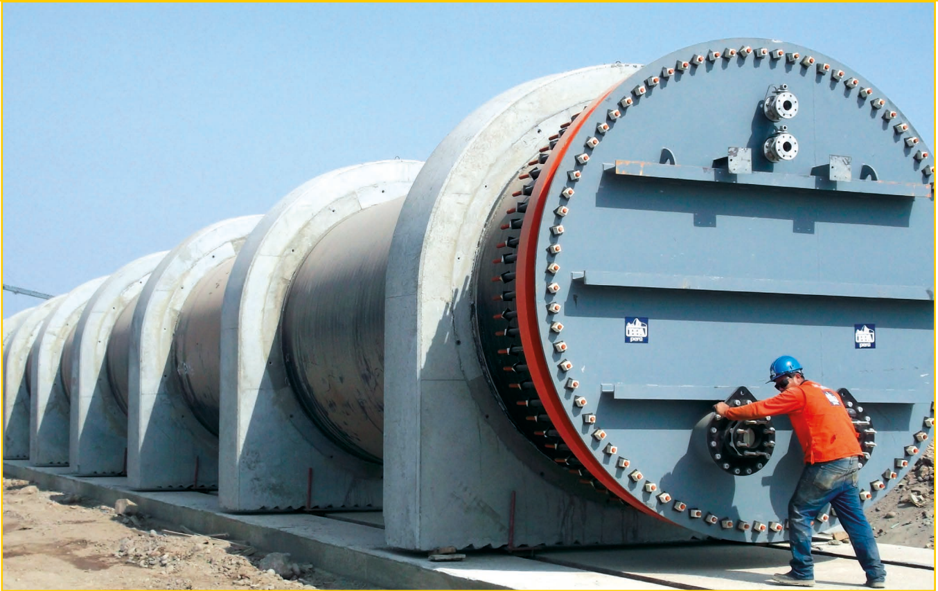
Preparing an outfall pipeline string DN/ID 3000mm (118")
