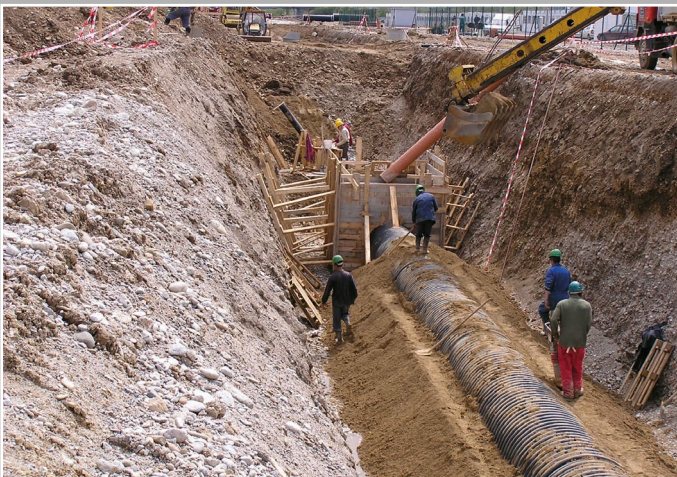
Installation of a sewage line DN/ID 1400mm (55") with a concrete manhole
