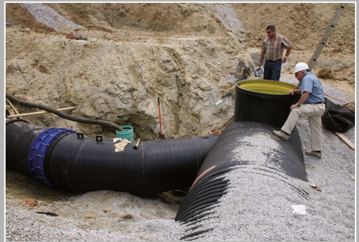
Installation of pipes DN/ID 2000mm (79"), with manhole & bench
