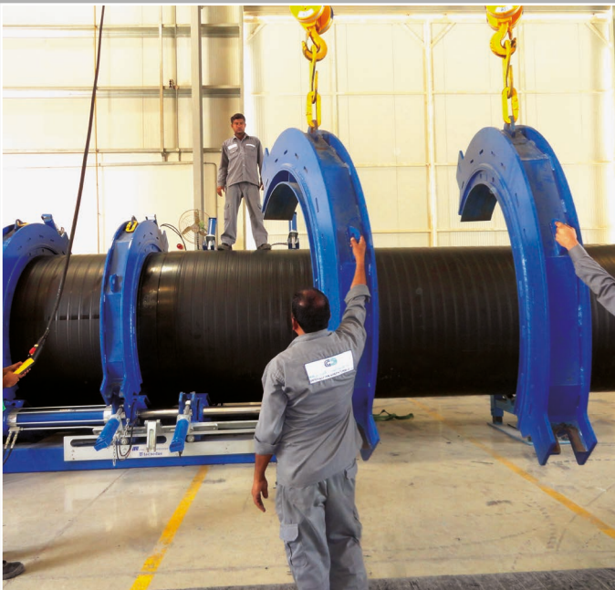
Butt-welding of pipes DN/ID 1800mm (71")
