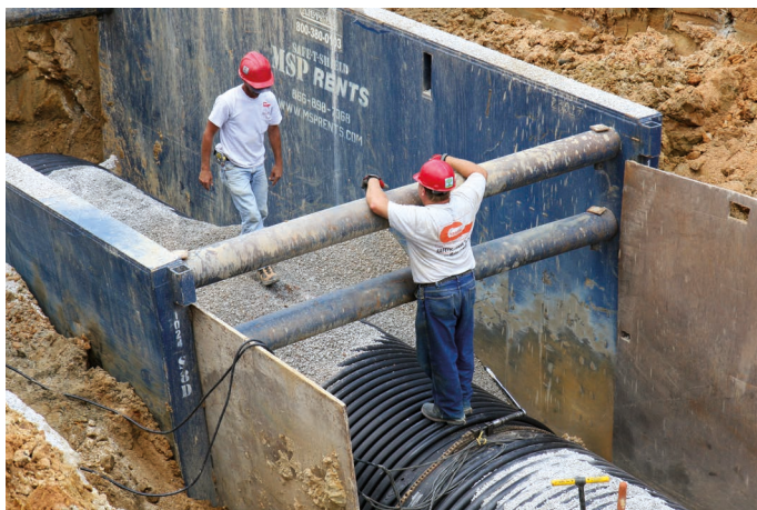
DN/ID 2200mm (87") pipe installation
