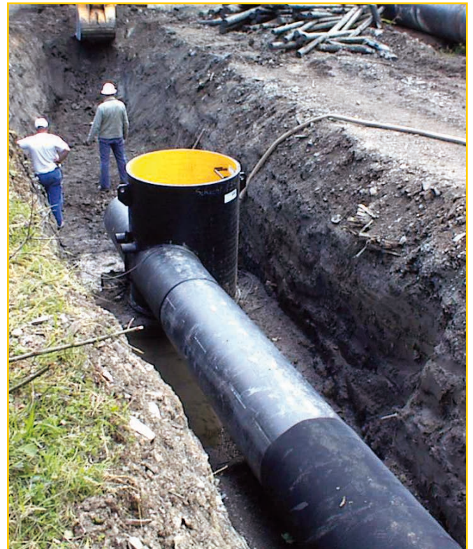
Installation of tangential manhole
