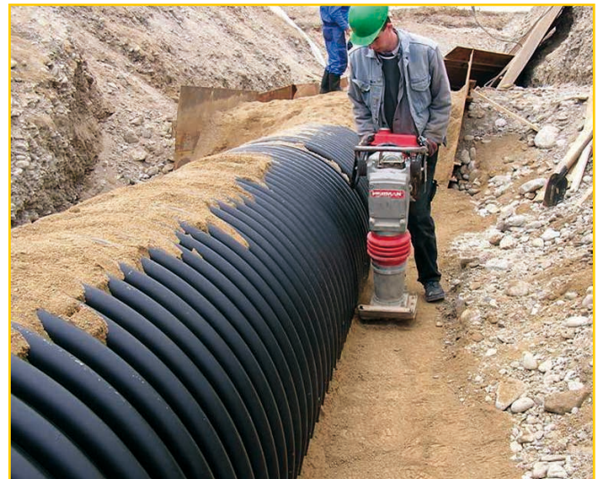
Compaction work with a vibratory plate
