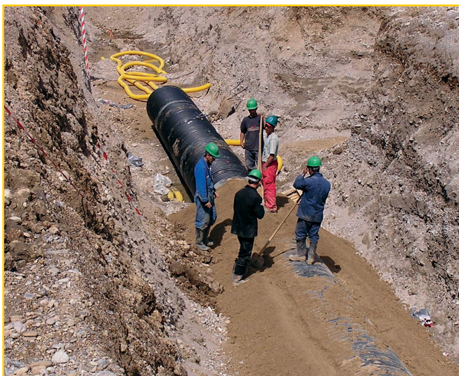
Compaction of main backfilling
