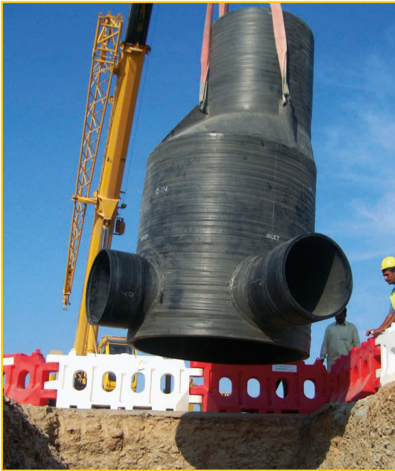
Manhole transportation on site
