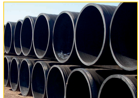
Storage on site
