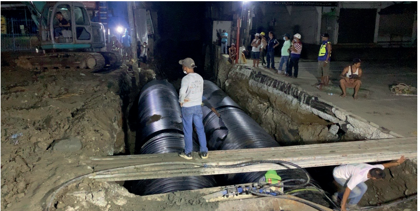
On-going installation of Krah structured wall pipes
