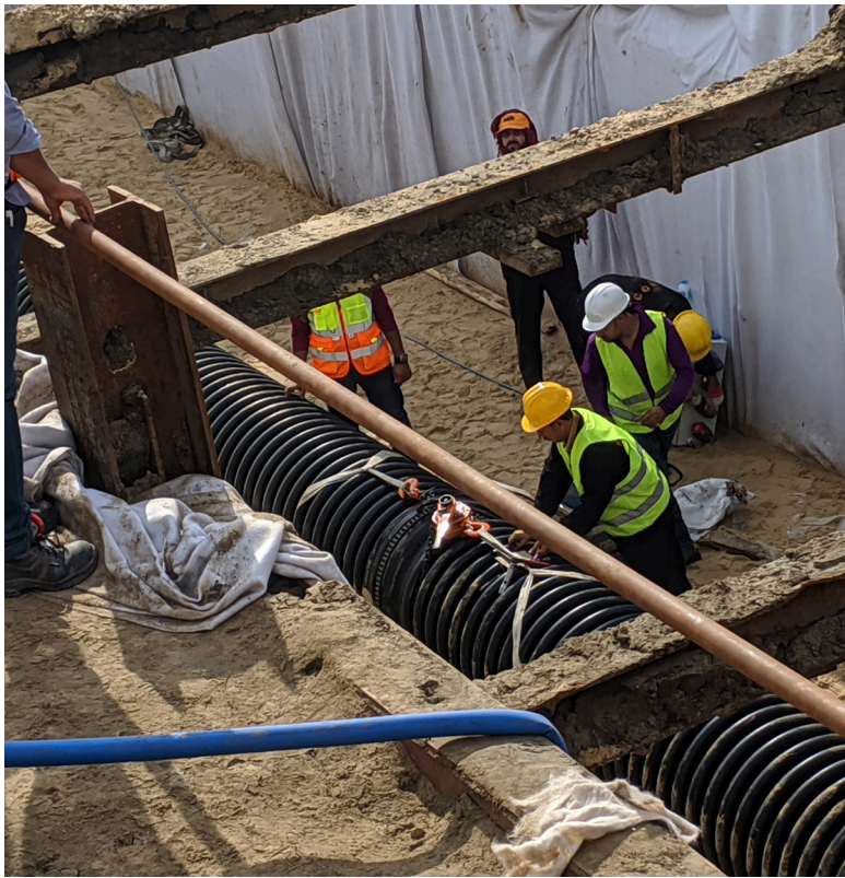
Krah pipes during installation
