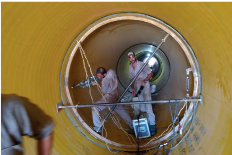
Welding under progress
