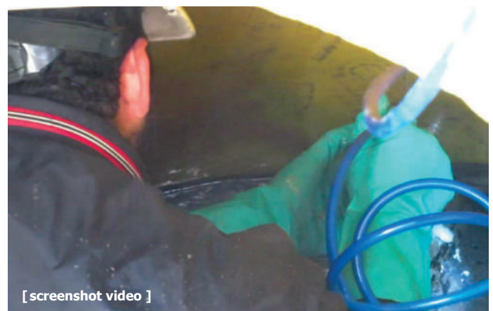
Manual welding of the broken part, after the infiltration is stopped
