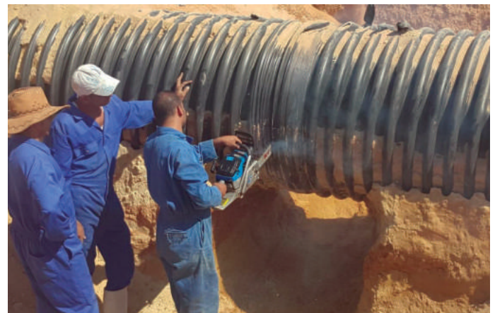
The broken pipe, is cut by a standard chain saw
