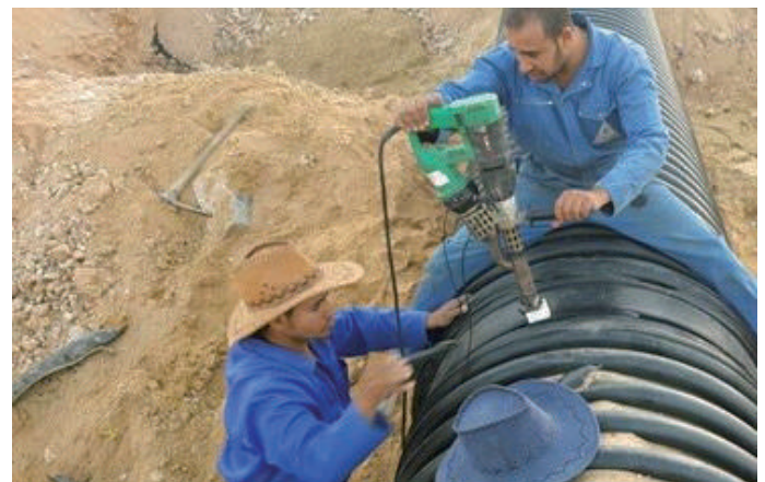
Manual welding under progress
