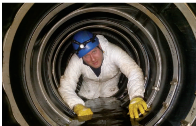
Worker inside the pipe, during installation of the Amex-liner
