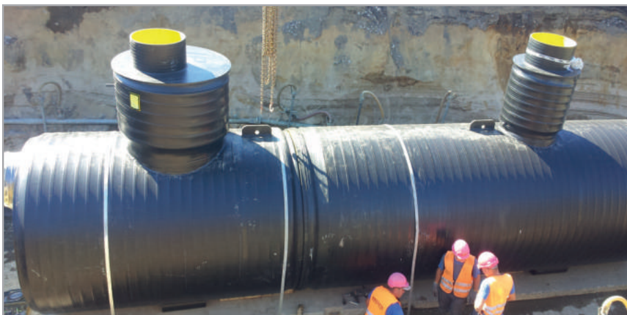
fig.4: Separator system at installation
