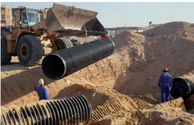
The new pipe will be placed
